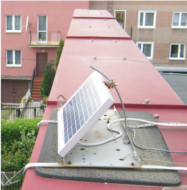
Fig. 1. Experimental solar module installation.
